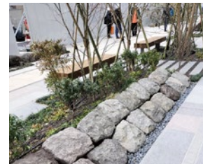
Stonework along Takanawa Link Line
